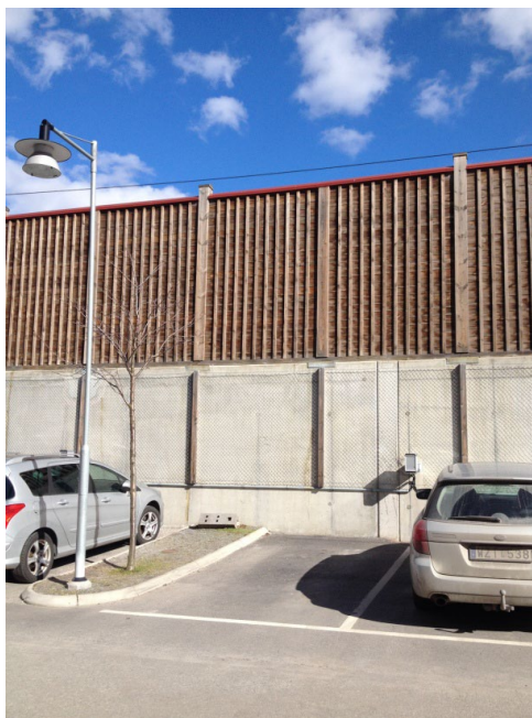
Fig. 2. A barrier protecting buildings from the noise of the high-speed railway. Sweden
